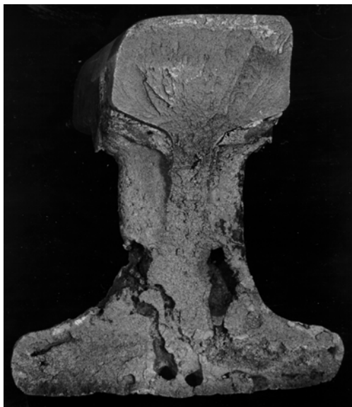
Figure 42: Fracture of an alumino-thermite weld due to weld defects in the foot.
